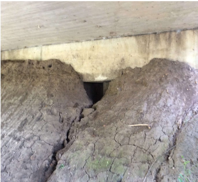
PHOTO 1 Description Bent 9 embankment erosion.
