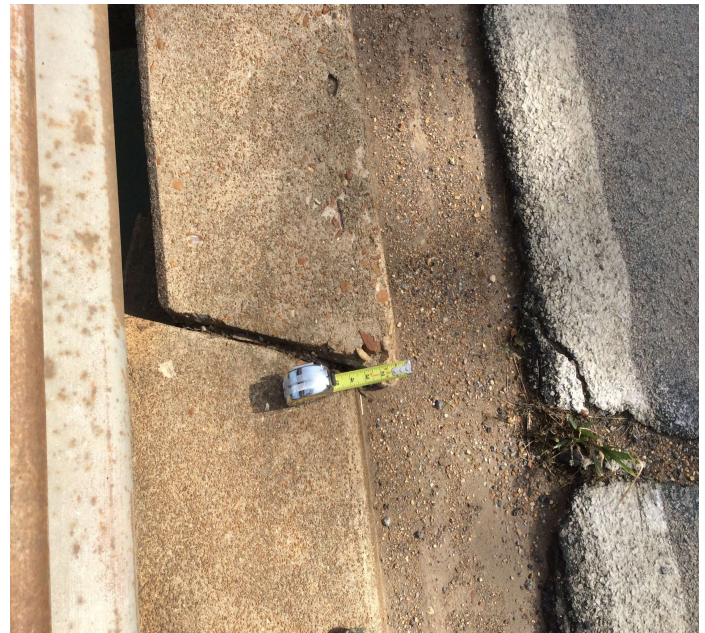
PHOTO 2 Description Bent 5 right curb lateral shift of slab.
